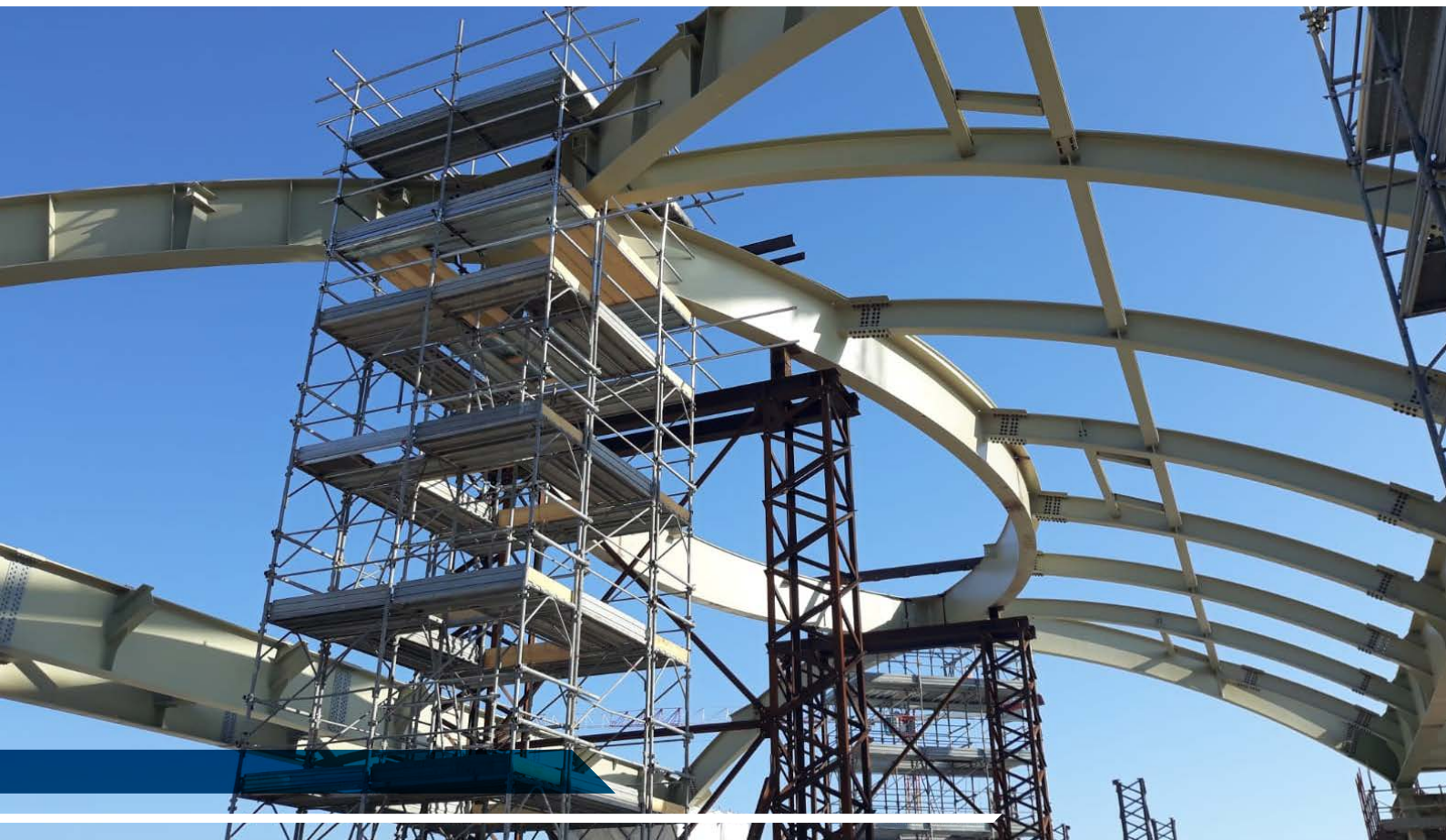
Roma Fiumicino Airport - Completion works for the land side and air side infrastructures of the East side terminal subsystem - Boarding area A, Terminal T1
